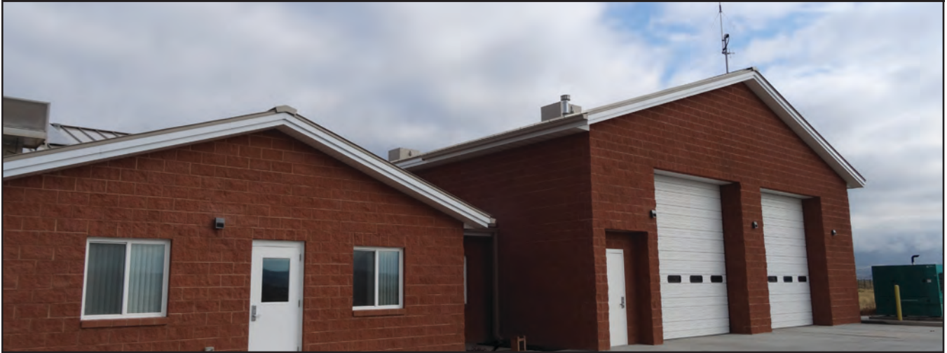
Figure 3.59 ARFF / Fire Station (27)
