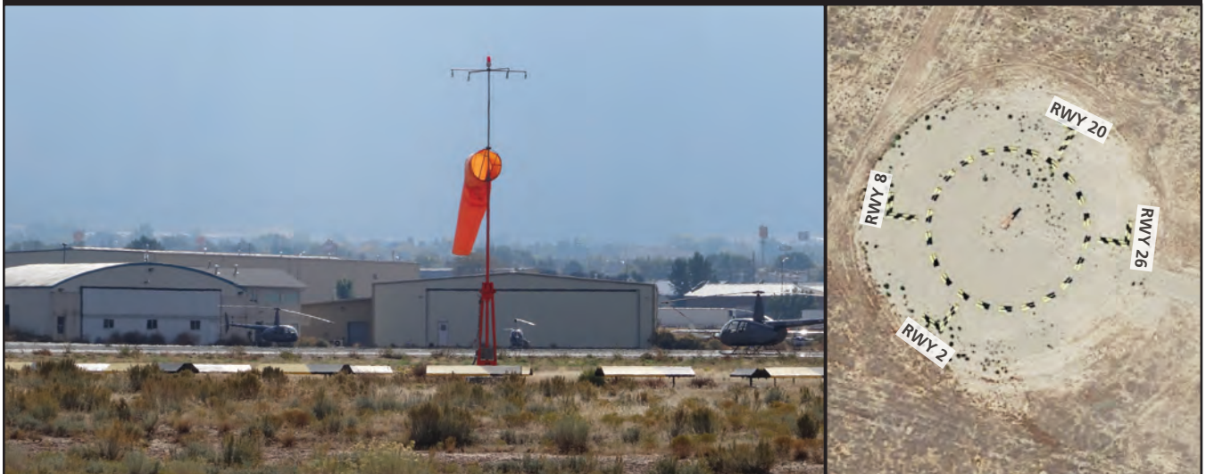
Figure 3.27 Segmented Circle and Primary Wind Cone (6)
