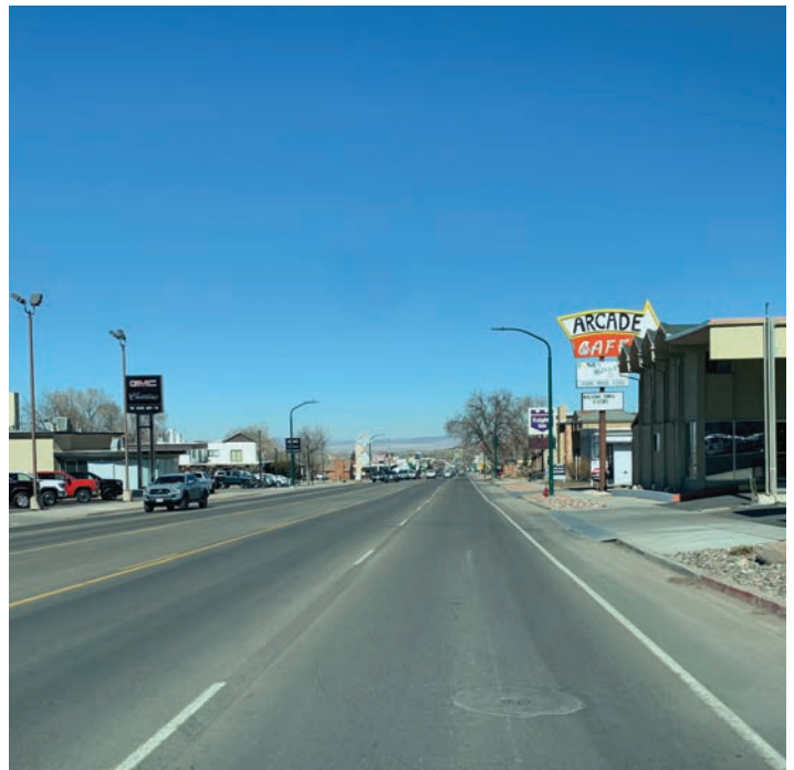
Figure 5-1. Main Street (SR-130) between 200 S & 400 S, a principal arterial in Cedar City.
